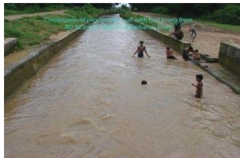
Renovated portion of Hirakud Distribution System
