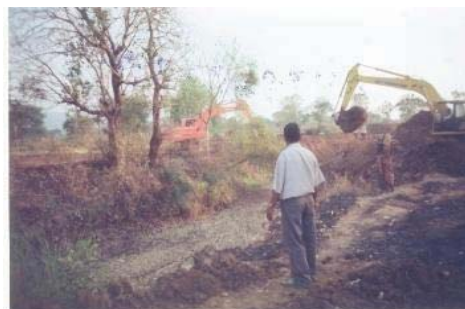
Kusumi Nallah excavation by excavator
