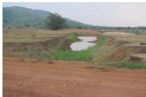
Incomplete Head Works
