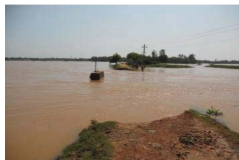
Breach at Gopaljewpatna
