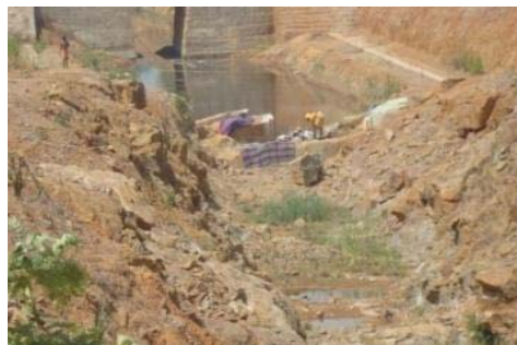
Incomplete Distribution System
