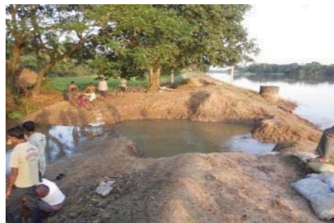
Breach in Double Embankment (right wing)
