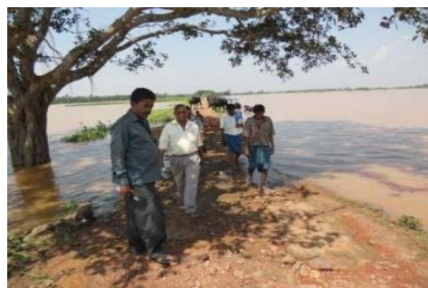
Overtopped Brahmani Left Embankment
