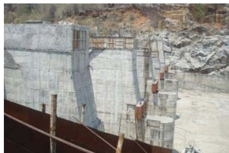
Incomplete Head Works
