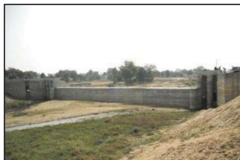
Completed Head Works of Chakramal MIP
