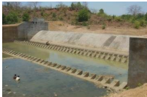
Completed Head Works of Saldihi MIP
