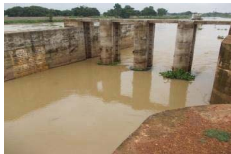
Incomplete Head Works
