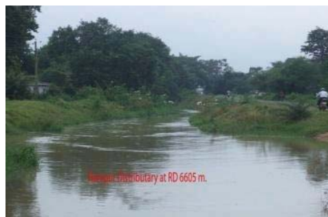
Eroded and unlined portion of Hirakud Distribution System not covered under RIDF
